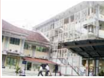
The main building of the school
